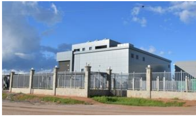
PHASE 2 DATA CENTER
