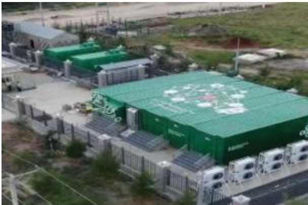
PHASE 1 DATA CENTER
